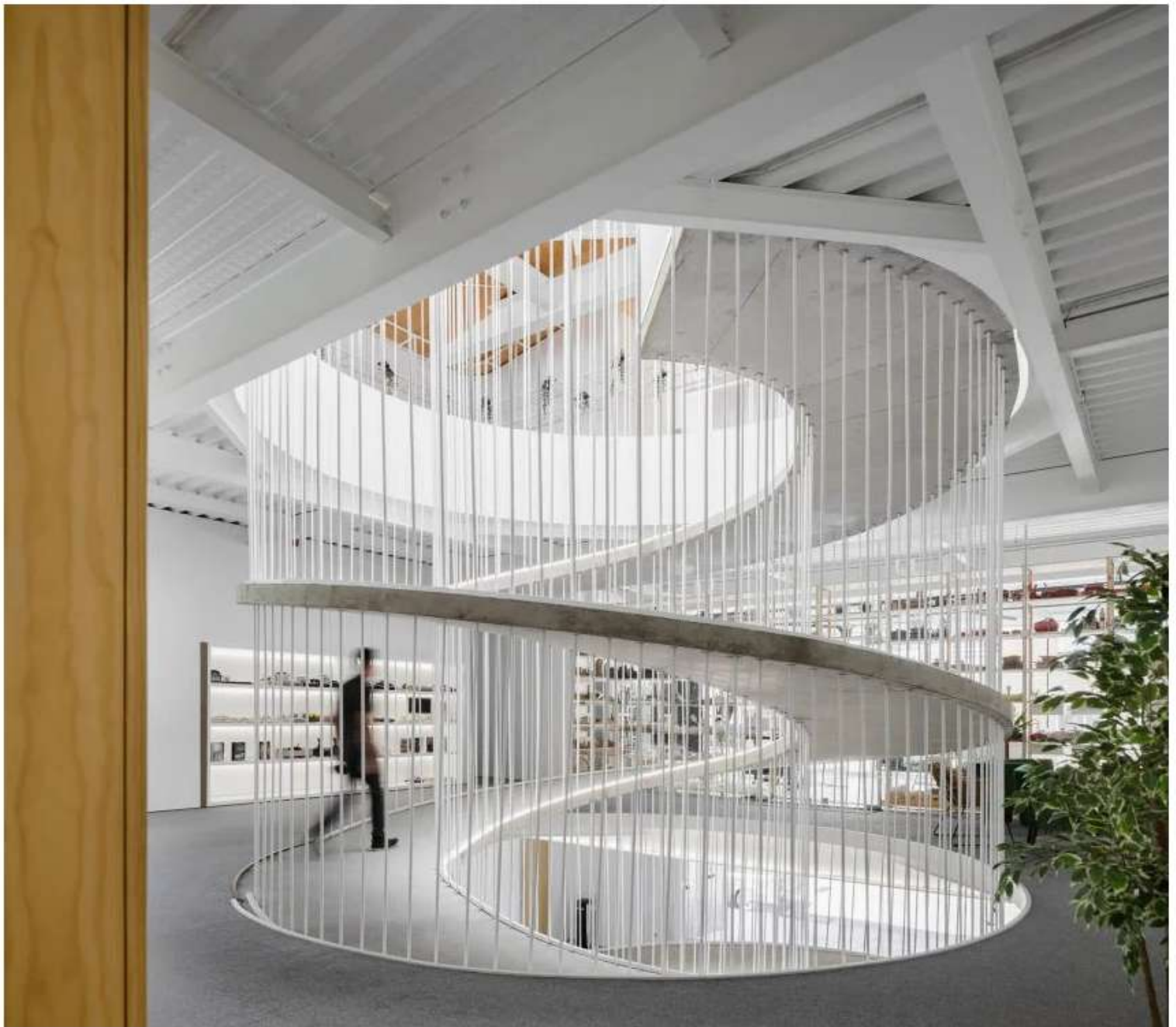
A spiralling concrete ramp connects the three floors
