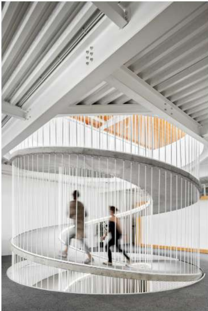
Above the ramp, a skylight was cut out of the corrugated aluminum ceiling.
