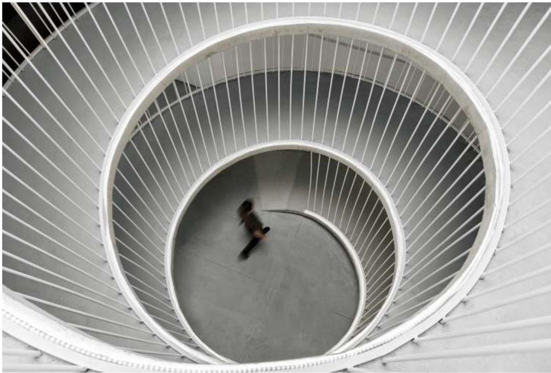
Lacquered iron tubes support the ramp from above as it winds through the office's three levels.
